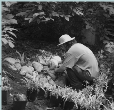
Constructing rain garden at Garden in the Woods
